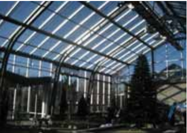
Company: Alberta Glass Project: The Zoo Conservatory Contractor: Ledcor Location: Calgary, Alberta
