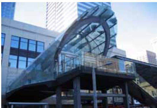
Company: Ferguson Glass (Western) Ltd. Project: 7th Avenue LRT Block G + 15 Location: Downtown Calgary, Alberta
