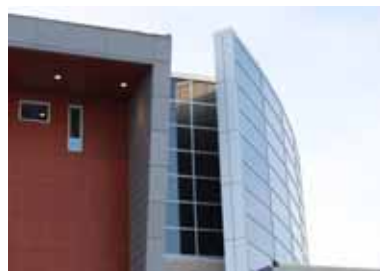
Company: Skyline Roofing Project: Glenmore Water Treatment Plant Product: Zinc, Prodema Panels Location: Calgary, Alberta General: PCL
