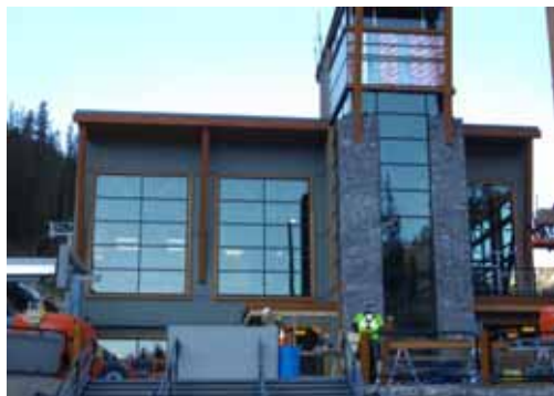
Company: DESA Glass Project: Sunshine Village Location: Sunshine, Alberta
