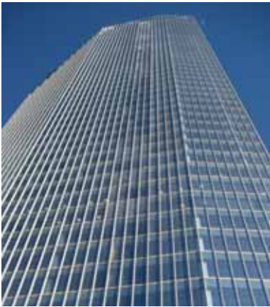
Company: Alberta Glass Project: Eighth Avenue Place Contractor: Ellis Don
